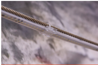
HALO Clips Installation
